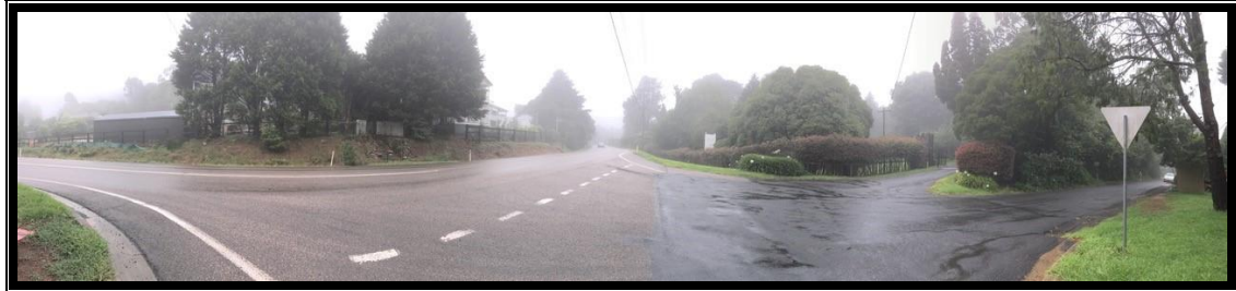
Photo 9: Adequate space between the exiting driveway and the Give-way line at Illawarra Highway
